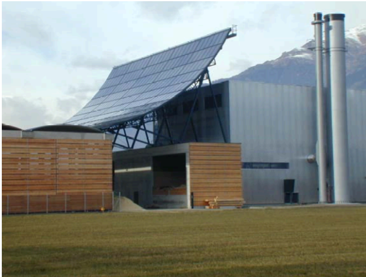
Biomass CHP plant based on an Organic Rankine Cycle process (Lienz, Austria)
