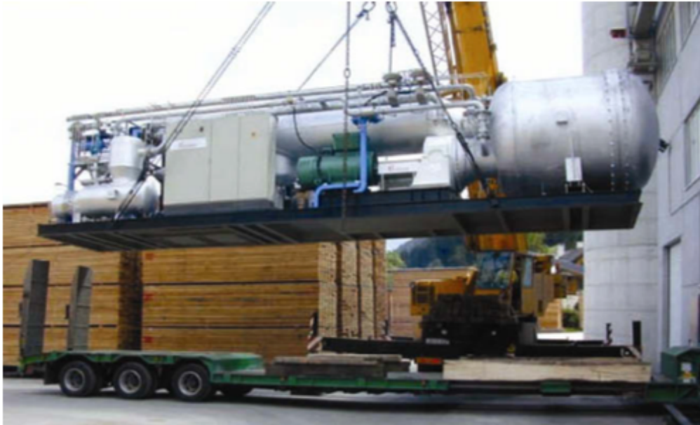
Overview of the whole module of the biomass-fired ORC Plant
